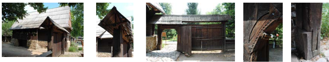
Fig. 5. Vernacular construction typology with round fir logs resting on a plastered stone foundation.
