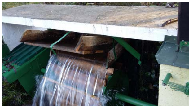
Fig. 9. Detail for turbine and equipment Turbine ongoing – The mobile spout is up.
