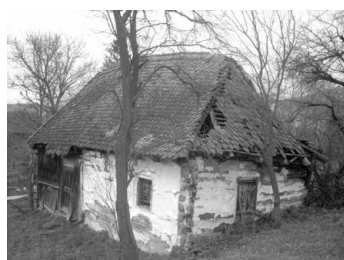
Fig. 1. House before demolition, 2000.
